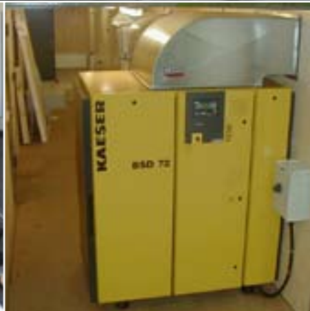
Switch house with panels and compressor
