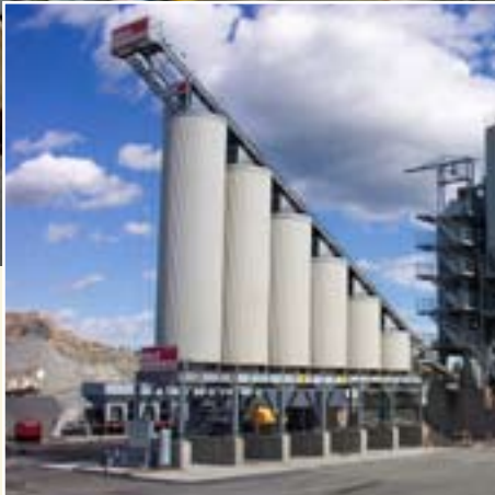
Cylindrical silos and inclined skip track
