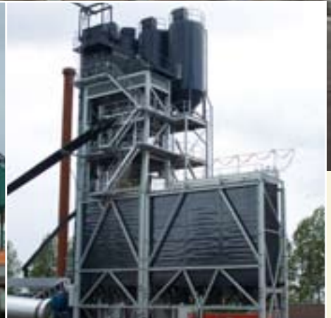
Square silos and horizontal skip track
